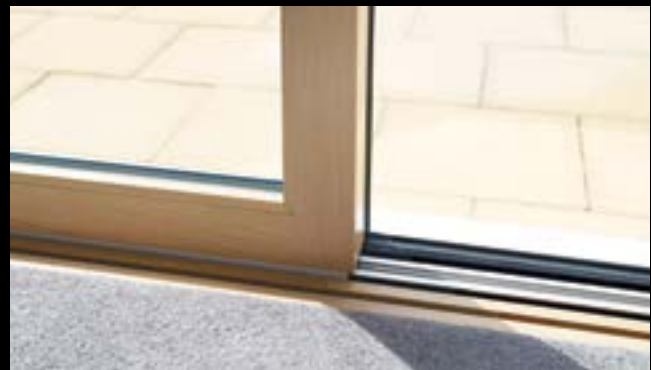
Sliding panel aligns with the mullion
